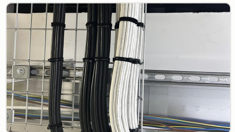
CONTAINMENT & RISER WORKS
